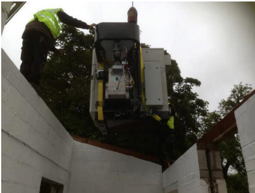
Ainscough Crane Hire lifting 199kW E-COMPACT in through roof of Plant Room
