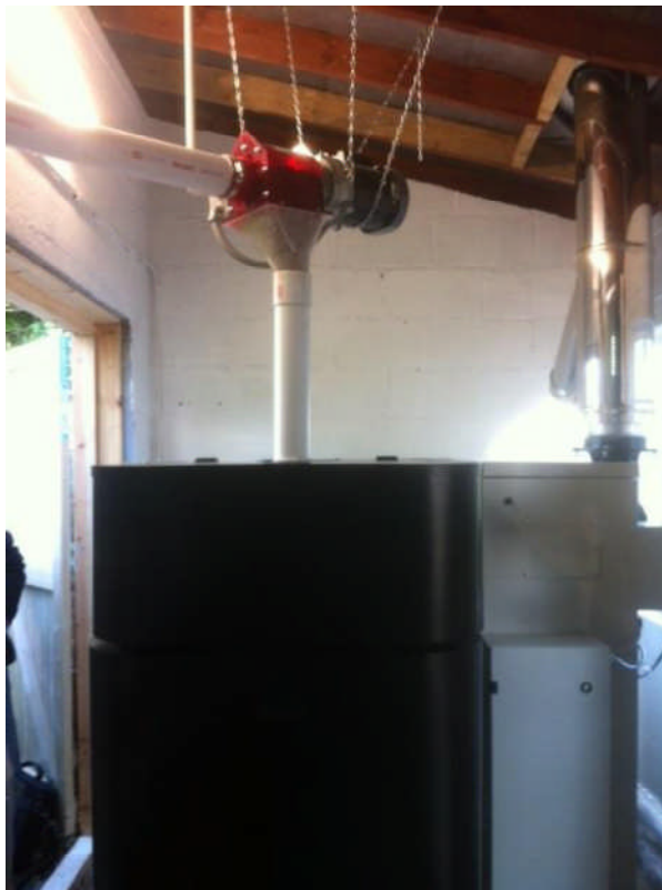
Auger Fed to 199kW E-COMPACT Pellet Boiler: Old Building converted to a Plant Room
